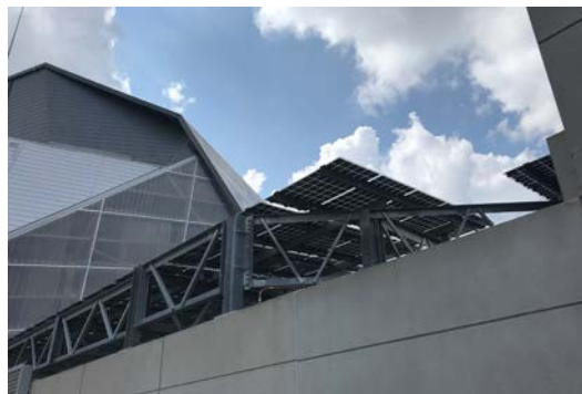
Figure 25. A solar energy system built atop the parking deck of the Mercedes-Benz Stadium in Atlanta, Georgia. 216
