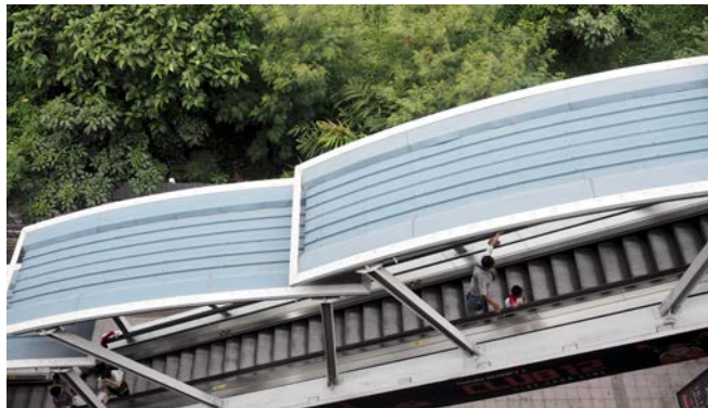
Figure 6. Solar canopies over an escalator. 21
